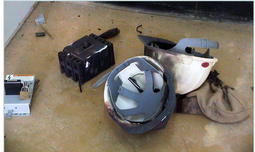
Figure 1-1. Breaker and hardhats on the utility room floor post-event
